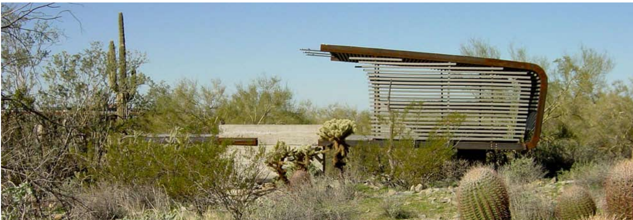
Hook Shelter, Scottsdale, AZ Luis Salazar, Taliesin West
