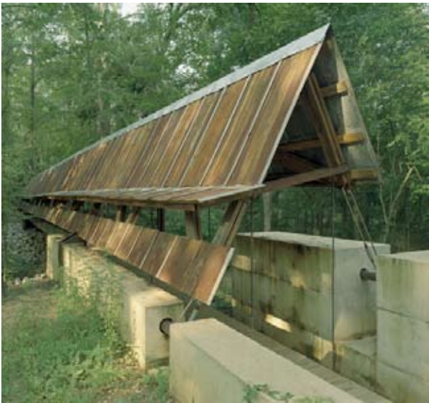
Perry Lakes Park Covered Bridge, Marion, AL Rural Studio
