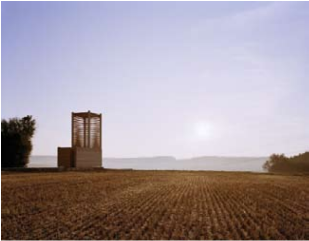
Field Chapel, Boedigheim, Germany Illinois Inst. of Technology & Ecker Architekten
